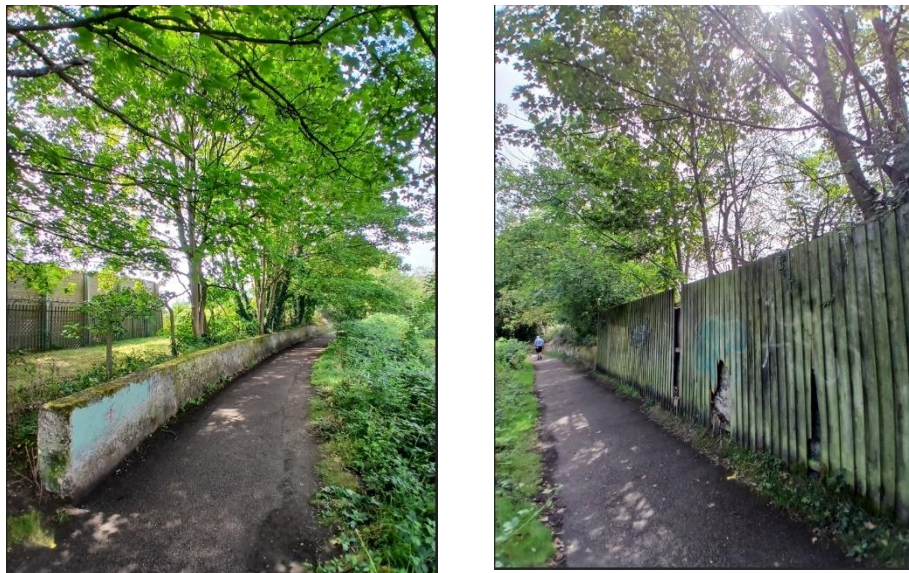
Figure 5 – Retaining Wall Structure. Images from Project Centre
